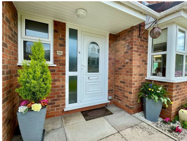
Outside light. UPVC double glazed entrance door to the entrance hall.
